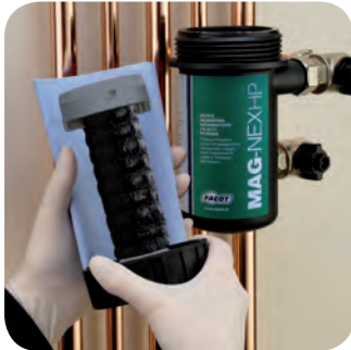
Figure 5 - Magnet impregnated of magnetic sludge
