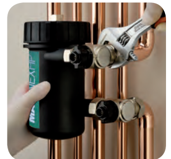
Fig. 3 - Tighten the compression joints
